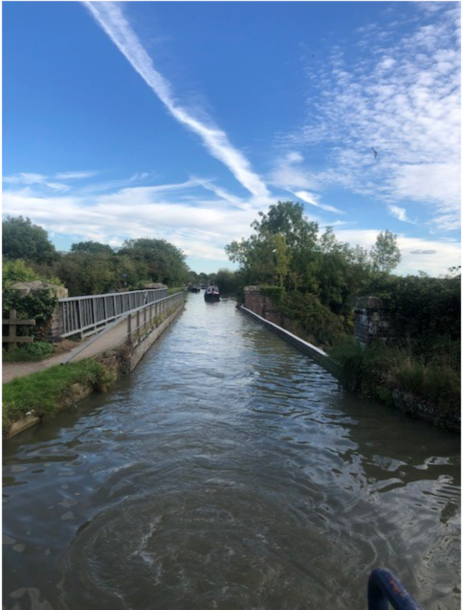
Cosgrove aqueduct is a navigable cast iron trough navigable aqueduct that carries the Grand Union Canal over the River Great Ouse, on the borders between Buckinghamshire and Northamptonshire at the northwest margin of Milton Keynes in England photo David Bellamy
