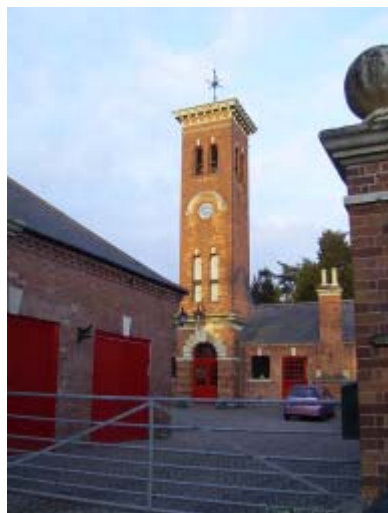
Gumley Hall Stables and clock tower.
